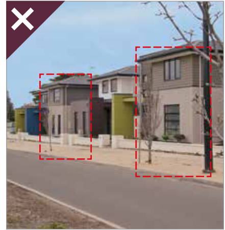
Example of non compliance façades, identical façades to close together.
