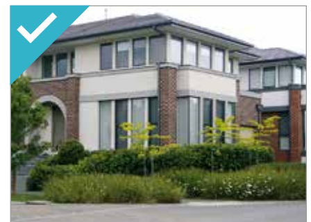
Example of compliant treatment, articulation of corner and verandah wrapping the corner.
