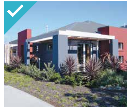
Example of compliant treatment, articulation of corner and verandah wrapping the corner.
