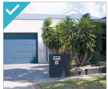
Example of compliant letterbox.
